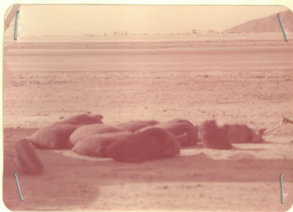
10 View of the Cargo removed from the aircraft on the 9th October, 1982. The Cargo of prawns were packed in gunny bags which were found to be soaked at the time of removal. The ground below the aircraft belly was also wet.
