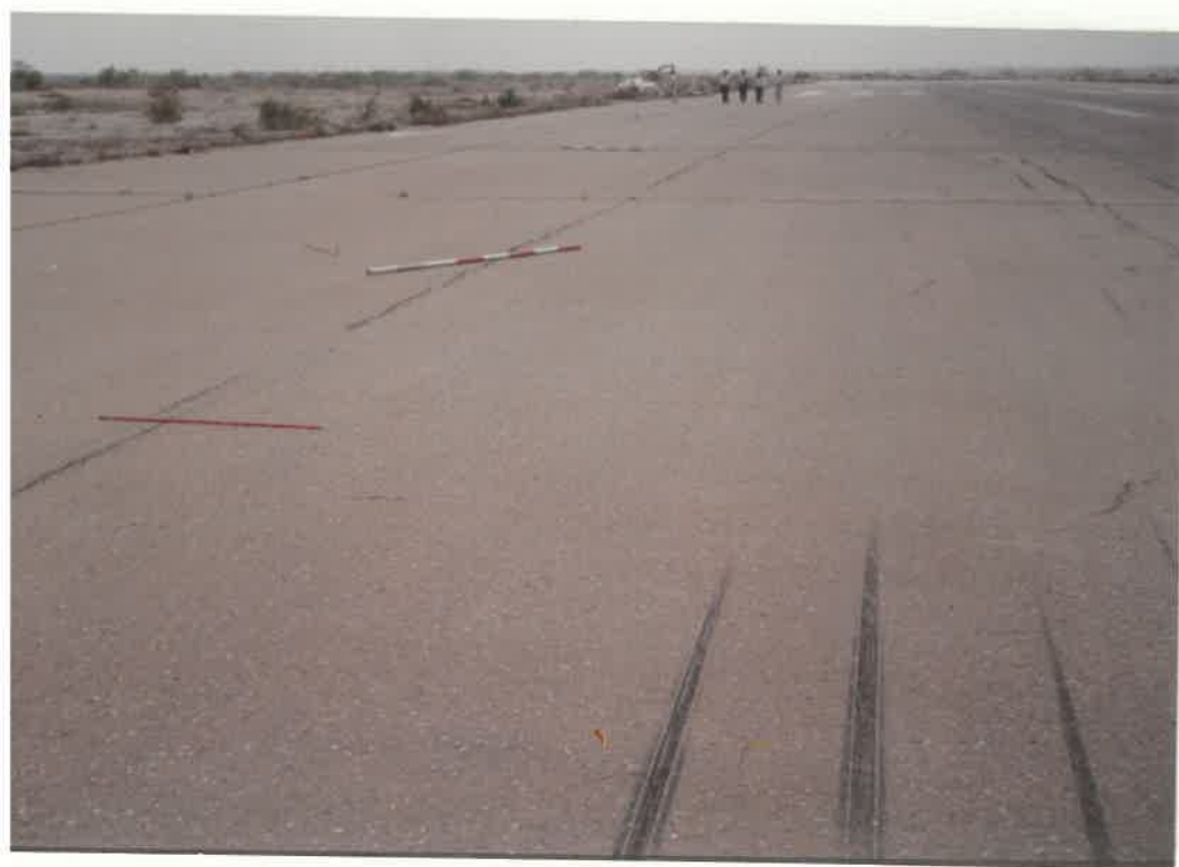
BARRICADE BROKEN PARTS.
