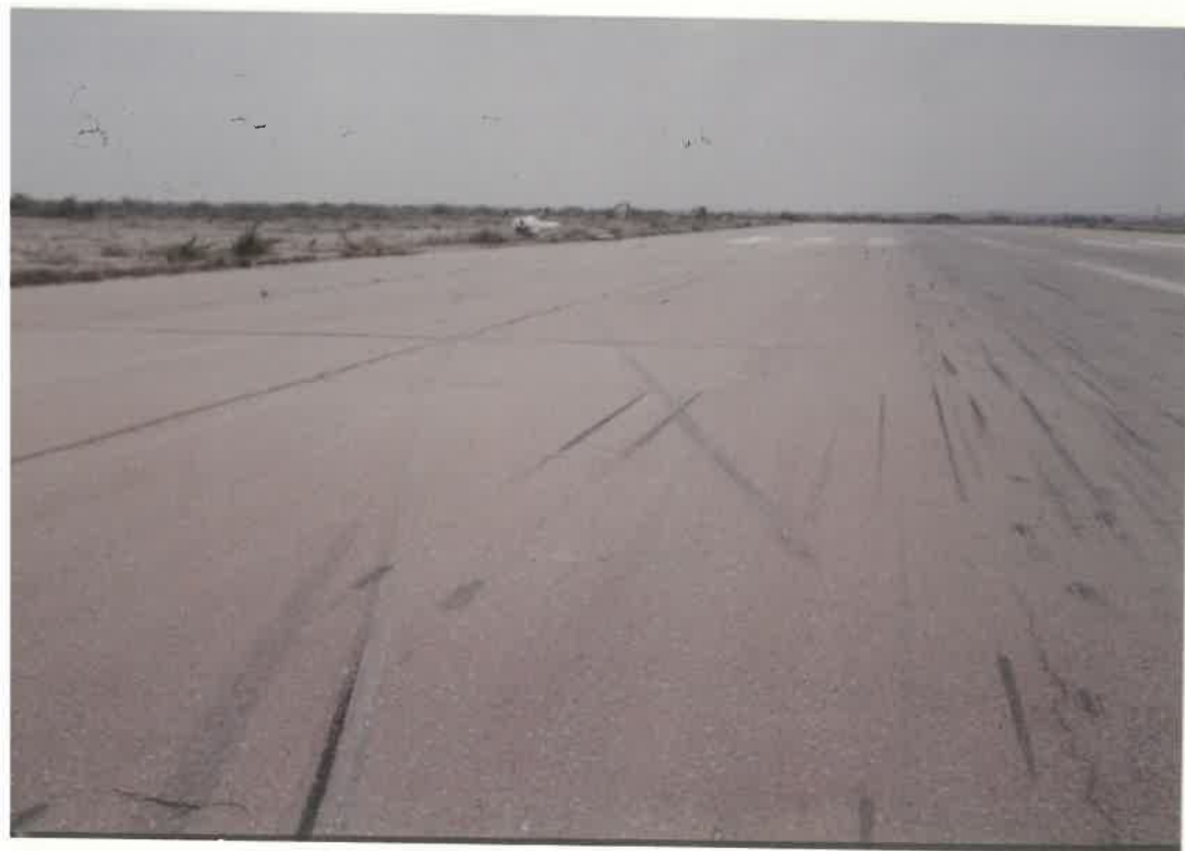
EVIDENCE OF TYRE MARKS ABOUT 180 FT FROM THE AIRCRAFT.
