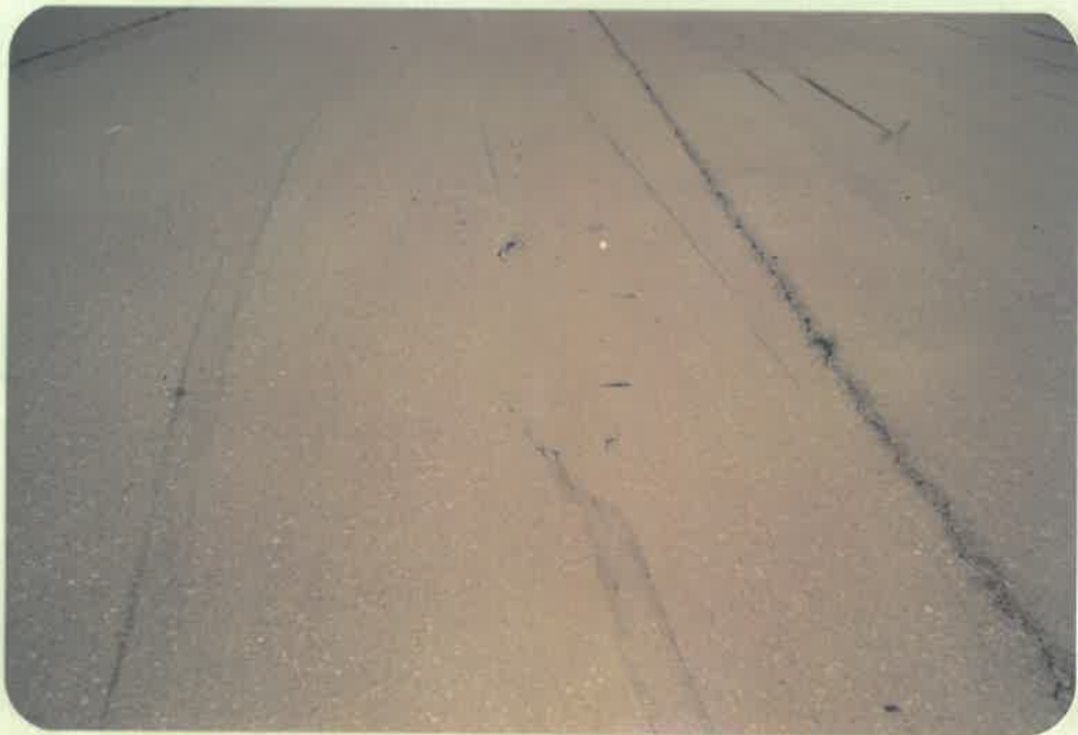
The track made on the runway after the nose wheel broke.
