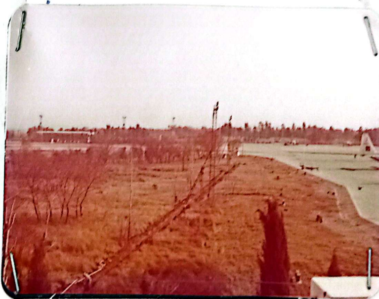
VIEW OF A PORTION OF TAXIWAY NO.1 AND APRON. FROM THE CONTROL TOWER. NOTE TAXIWAY NO. 1 OBSCURED BY TREES.
