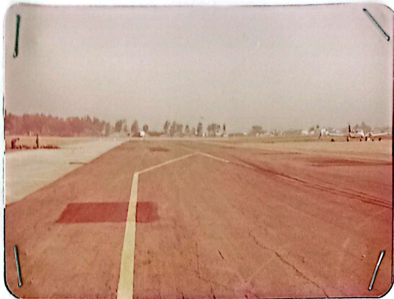
3 TAXIWAY NO. 1 INTER SECTION WITH RUNWAY. THIS VIEW SHOWS THE OFF SET CENTRE LINE AS SEEN FROM APRON.
