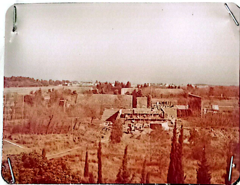
6 VIEW OF MANOEUVRING AREA FROM THE CONTROL TOWER.
