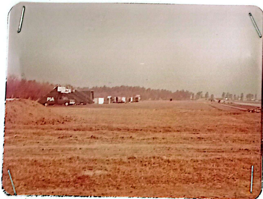
HARDSTAND FOR M/S. P.I.A.C. GROUND EQUIPMENT. THIS IS WEST OF THE TAXIWAY AND RESULTS IN GROUND EQUIPMENT CROSSING THE TAXIWAY TO PROCEED TO AND FROM THE APRON. THIS IS UNDESIRABLE SINCE IT CAN BE A CAUSE OF FOREIGN OBJECTS ON THE TAXIWAY/APRON.
