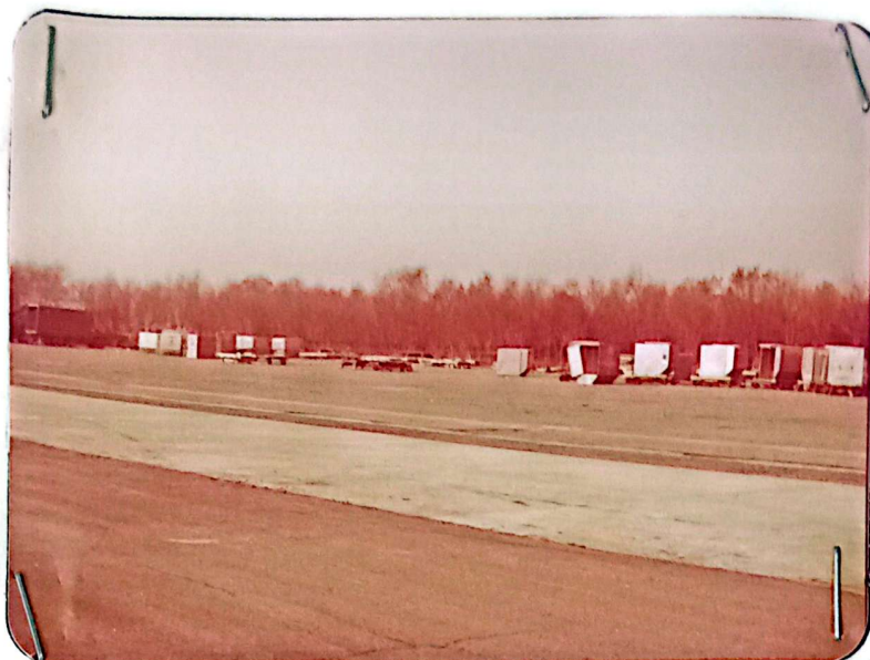
5 VIEW OF CONTROL TOWER FROM TAXIWAY ONE. NOTE ONLY TOP OF THE A.T.C. BUILDING CAN BE SEEN.
