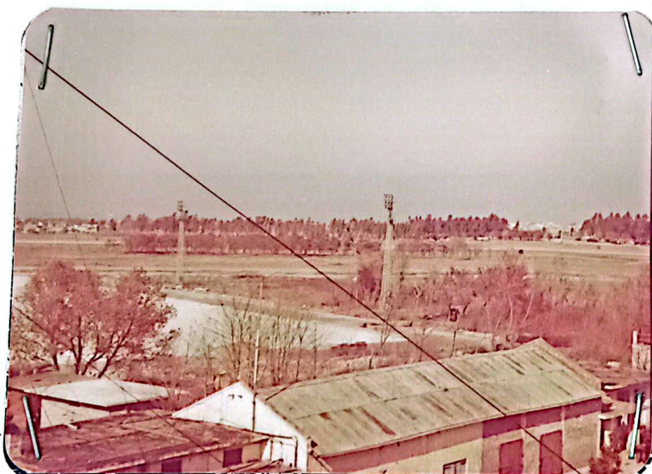
VIEW OF 1ST 2000 FEET OF RUNWAY 30 TAXIWAY NO.1 AND 2. FROM THE CONTROL TOWER.
