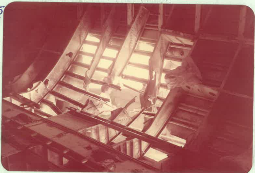
Damaged fuselage seen from inside.
