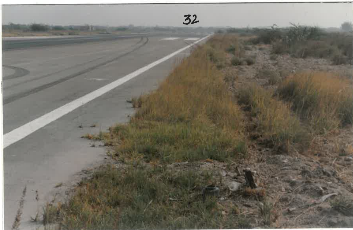
A/C LEAVING PREPARED SURFACE AT 1150 FEET FROM THRESHOLD R/W 32
