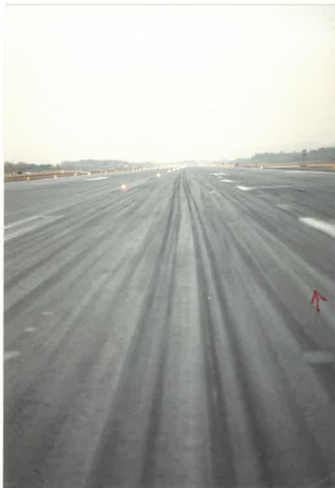
TYRE MARKS OF RT MLG TYRES ABOUT 2000 TO 3000 FEET FROM THE STOPPING POINT OF A/C.
