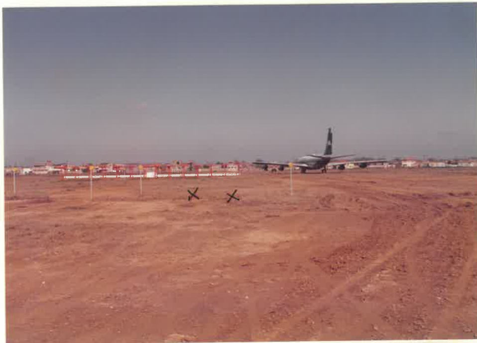
TWO APPROACH LIGHTS MISSING AND DEPICTION OF CLOSENESS OF THE AIRCRAFT TO THE BUILTUP AREA AHEAD (ONLY 500' TO 600' AWAY ).
