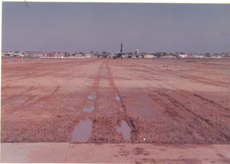
LEFT WHEEL TRACK ON KATCHA
