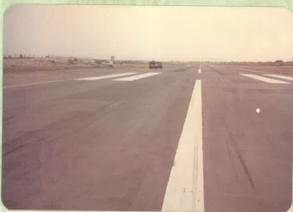
TYRE TRACKS SHOWING AIRCRAFT SWING TO THE LEFT.
