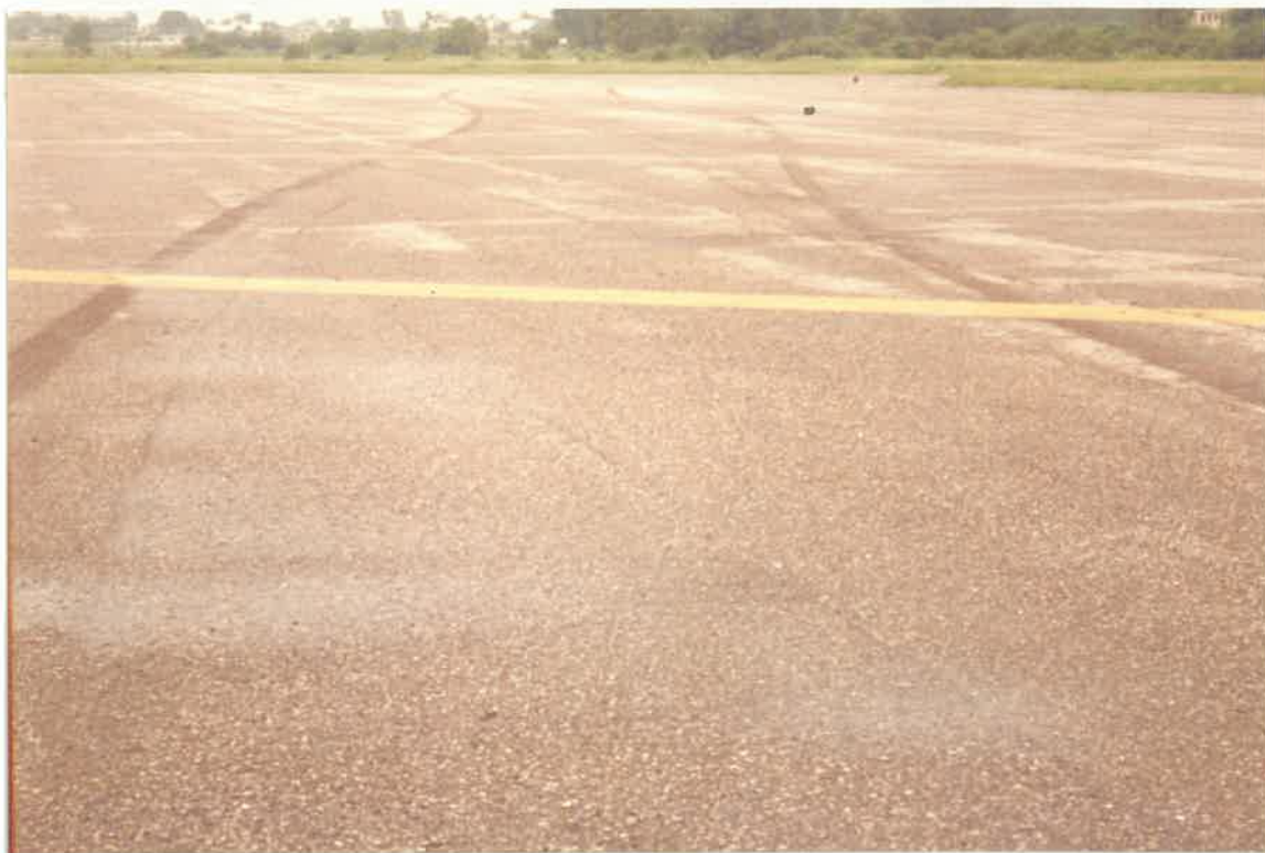
Both main landing gears wheels (outer only) marks upto end of over-run area.
