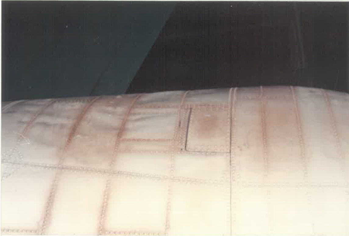
EVIDENCE OF BUCKLED TAIL SKIN DUE TO HEAT
