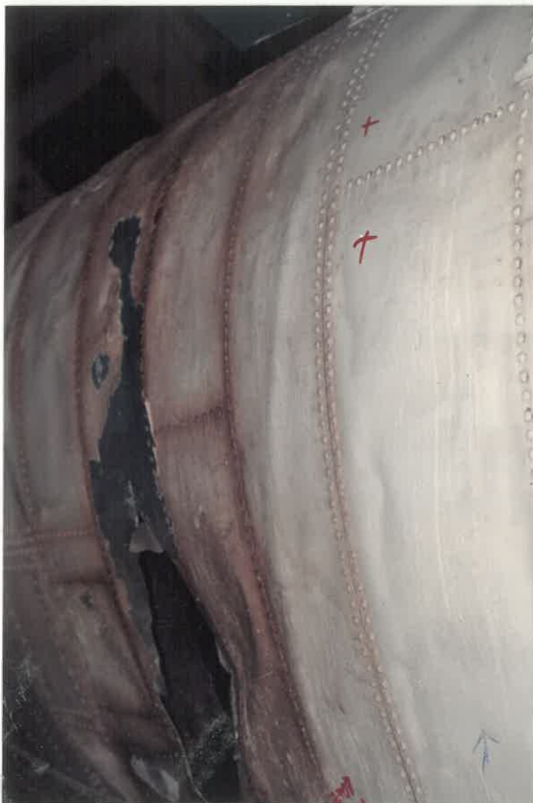
EVIDENCE OF BURNING AND BUCKLING OF TAIL SKIN
