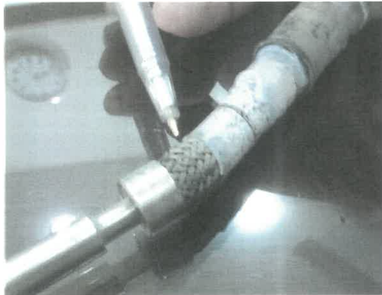
Location of the leakage on PB Line
