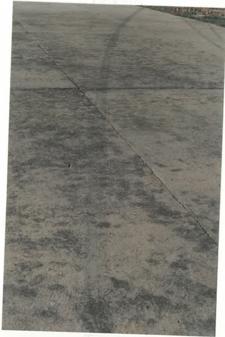
HARD BRAKE APPLICATION MARKS
