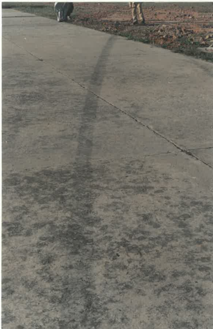
HARD BRAKE APPLICATION MARKS
