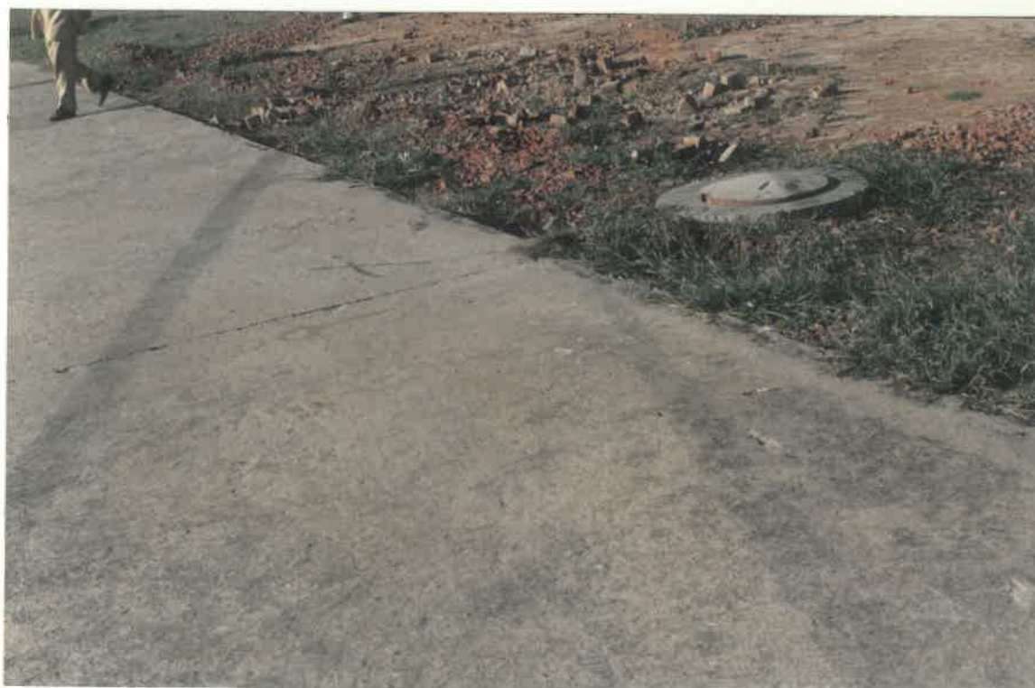
HARD BRAKE APPLICATION MARKS
