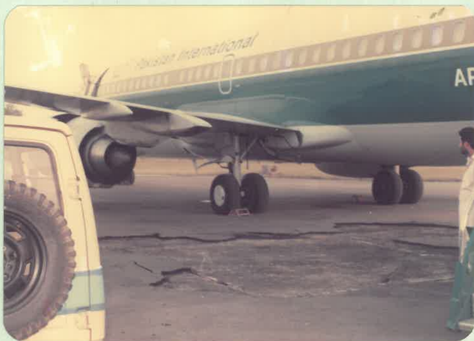
VIEW FROM THE LEFT SHOWING PEELED OFF OVERLAY ARROW POINTS MELTED BITUMIN
