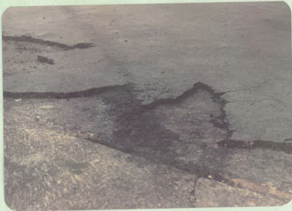
THIS VIEW SHOWS THE MELTED BITUMIN. SHOWN AT APPENDIX "B 2 "
